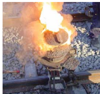
Welding railroad track with Thermite
